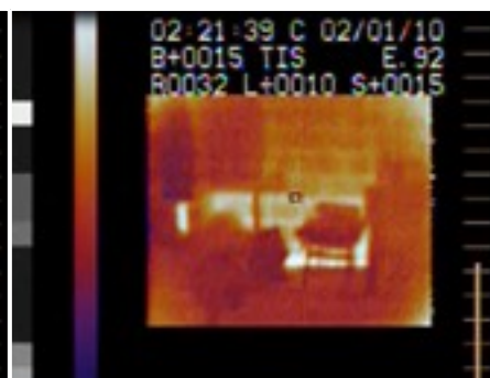
HEAT ESCAPING INTO GARAGE
